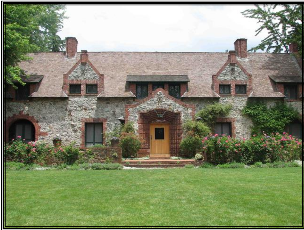
Bourn Cottage - Empire Mine State Historic Park Grass Valley
