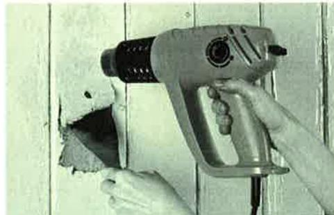
These work places will eliminate dust, but some renovation methods make less dust than others. Contractors may choose to use various methods to minimize dust generation, including using water to mist areas before sanding or scraping; scoring paint before separating components; and prying and pulling apart components instead of breaking them.
