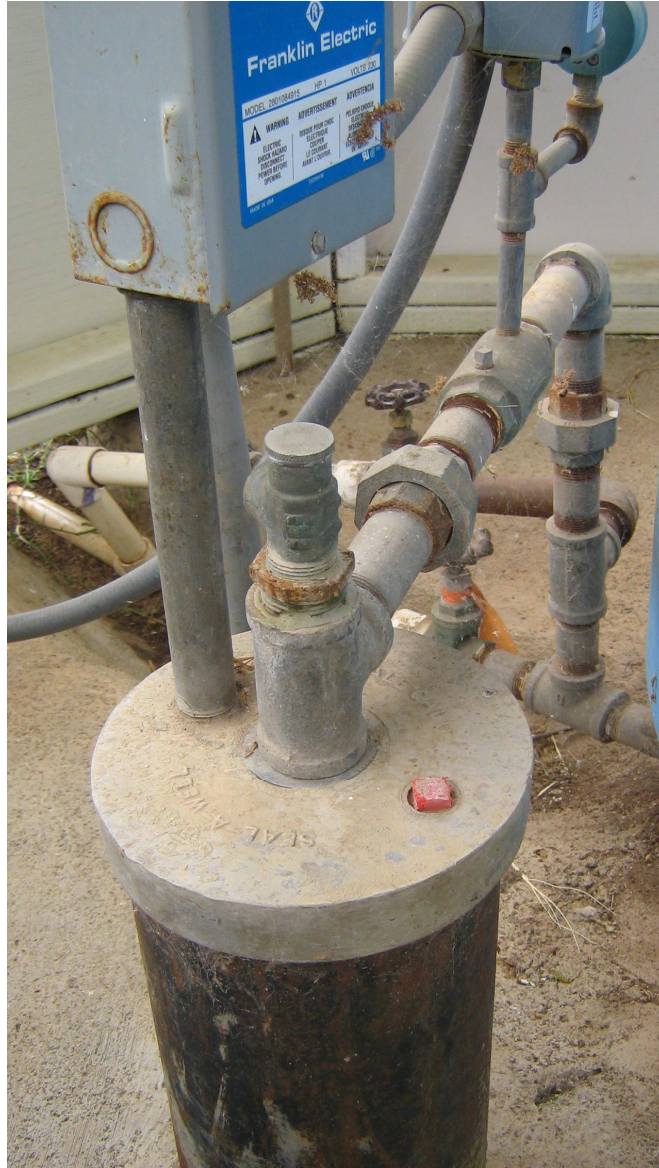
Photo: A domestic well showing the well casing, cover, and conveyance system. The well is located inside a shed with a concrete floor.
