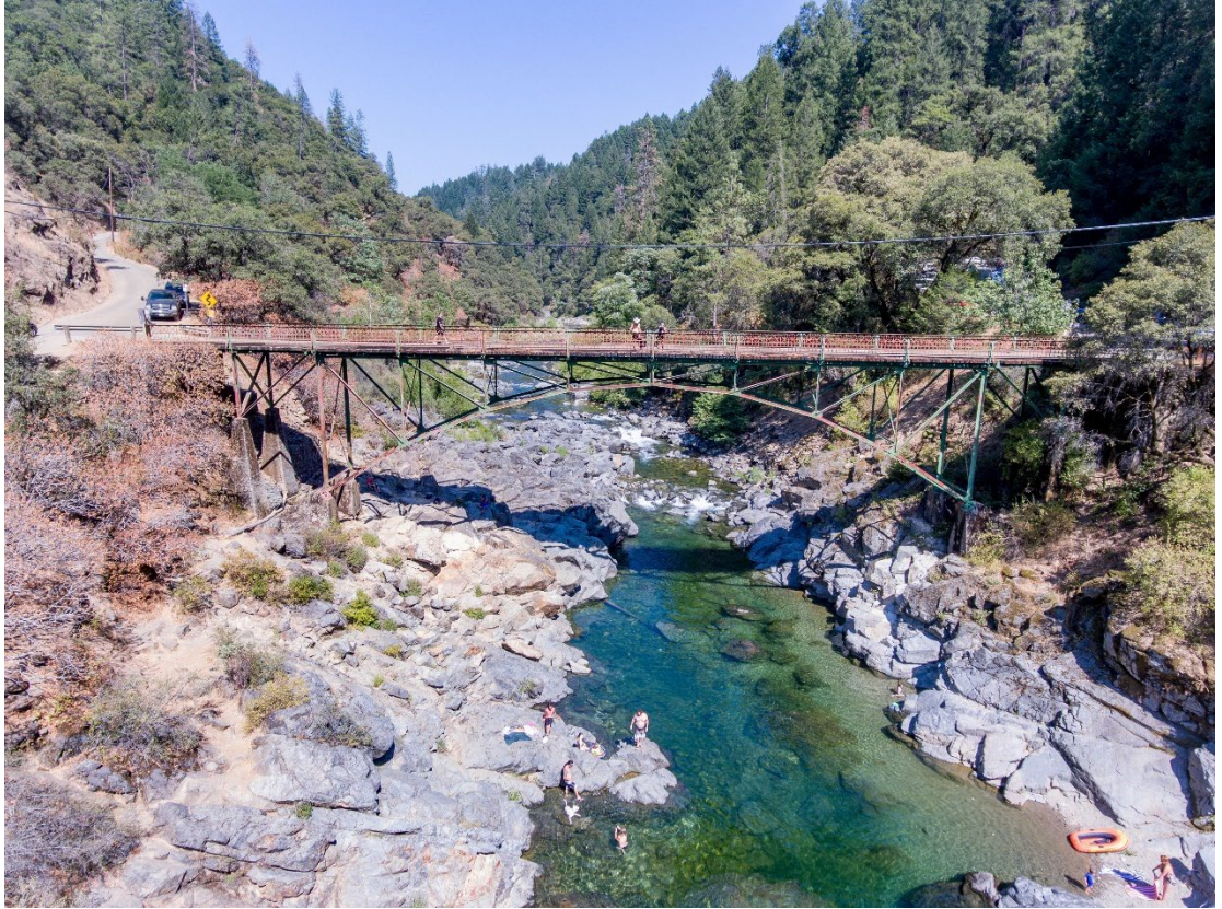
Edwards Crossing Bridge
