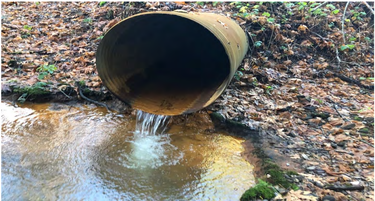
Photo 8: Existing culvert daylights within the Brunswick Industrial Site at the South Fork Wolf Creek just upstream from Photo 7.
