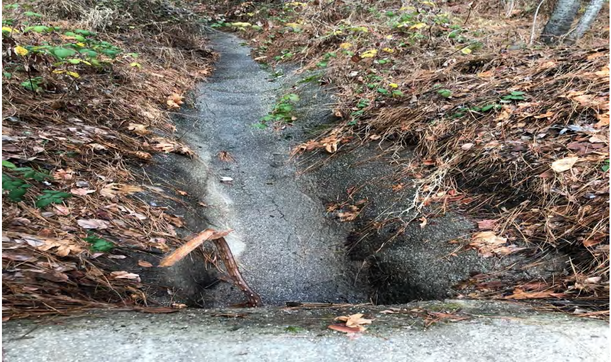
Photo 23. Manmade drainage along north side of East Bennett Rd. ROW. Drainage located outside of ROW and drains to the south side of East Bennett Rd. ROW.
