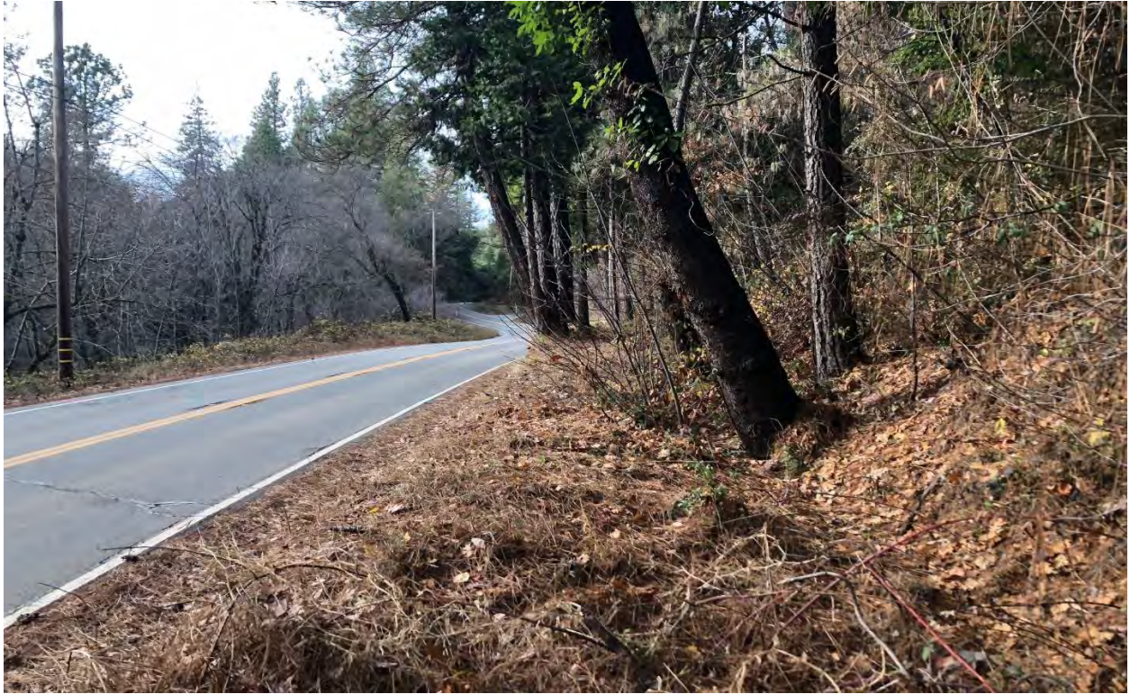
Photo 25. Non-jurisdictional roadside swale along northern side of E. Bennett Rd. ROW
