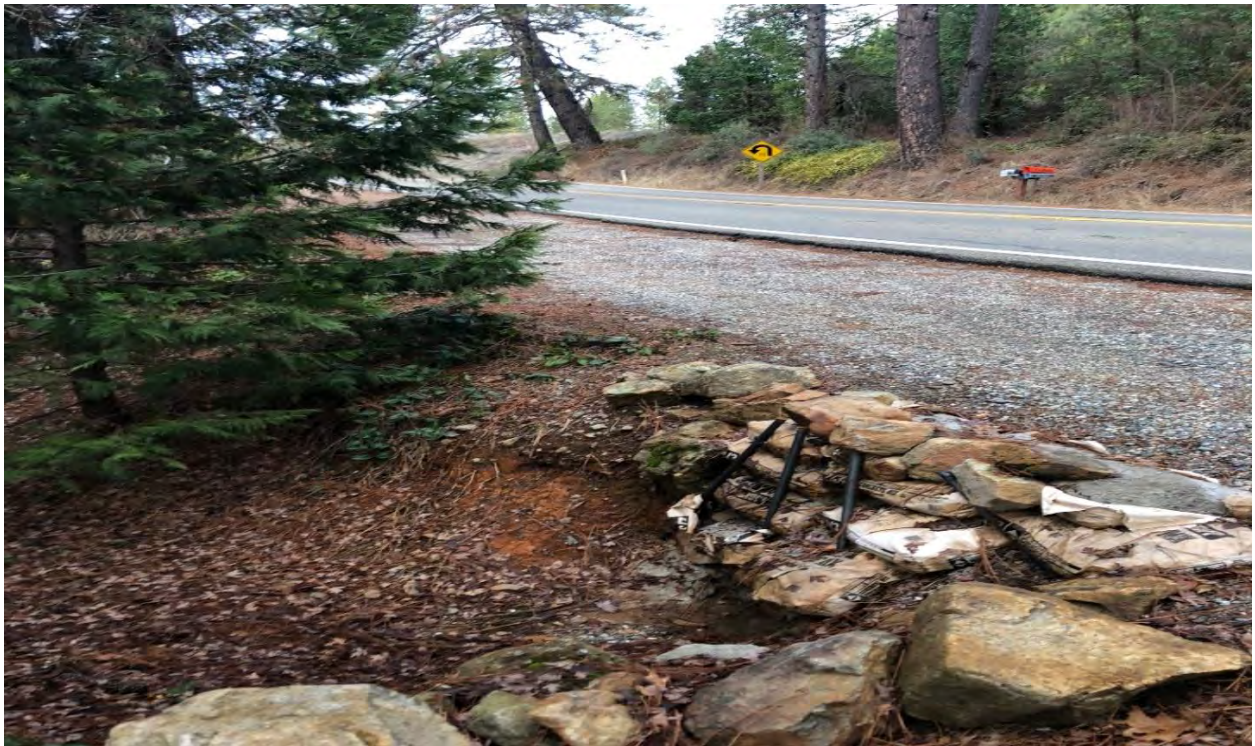
Photo 26. South side culvert/drainage along East Bennett Road ROW. Located towards lower end of E. Bennett Road ROW and within the developed part of the ROW.
