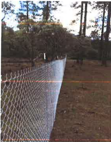
6' chain link boundary security fencing.
