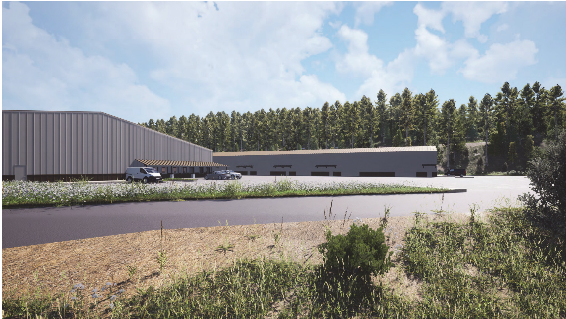
1 OFFICE & WAREHOUSE (SOUTH)
